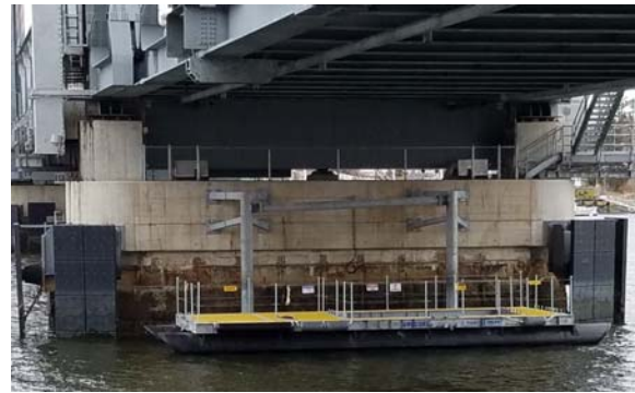
FIGURE 5. TURBINE DEPLOYMENT PLATFORM (TDP) DEPLOYED ON VERTICAL GUIDE POSTS, PIER NO. 2 AT MEMORIAL BRIDGE IN PORTSMOUTH, NH (MARCH 2017).
