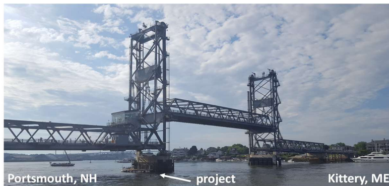
FIGURE 1. MEMORIAL BRIDGE BETWEEN PORTSMOUTH, NH, AND KITTERY, ME (LOOKING NNW). TIDAL ENERGY CONVERSION PROJECT/TEST SITE LOCATION IS ON PORTSMOUTH-FACING SIDE OF PIER #2.
